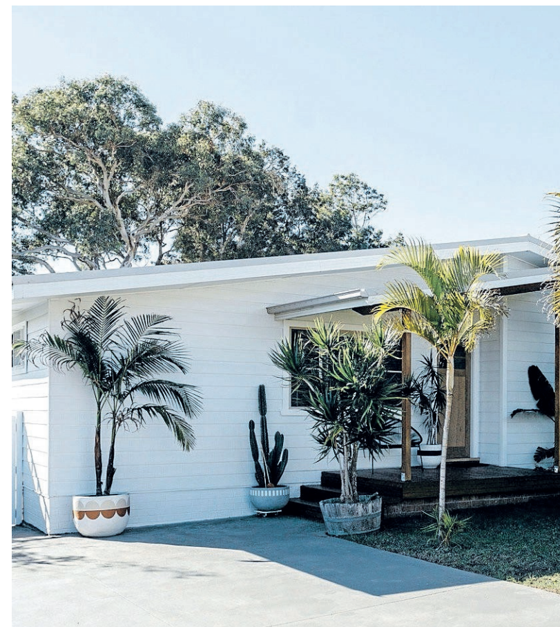
FRESH LOOK: Colorbond roofing and Weathertex cladding.
